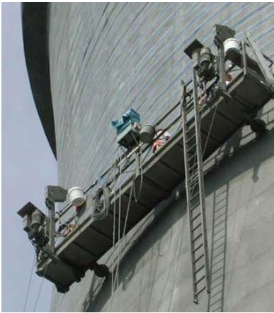
Winding the SikaWrap®-200 C carbon fibre reinforced fabric (width: 15 cm), centre-to-centre distance 30 cm.
