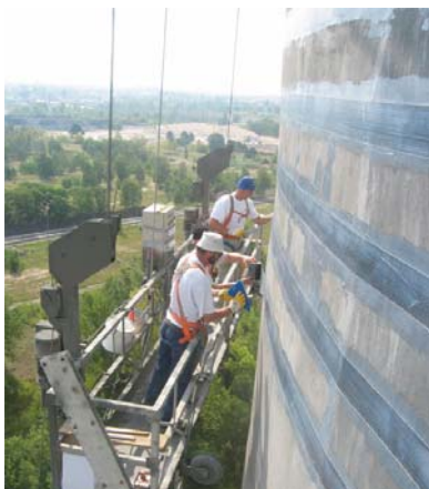
At a circumference of 120 m (bottom) and 70 m (waist), each wrap has at least 2 lap joints with a horizontal offset > 1.5 m.
