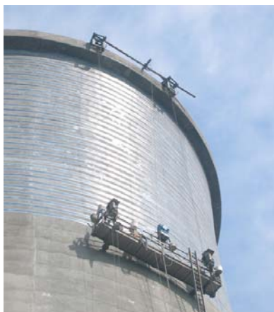
At a circumference of 120 m (bottom) and 70 m (waist), each wrap has at least 2 lap joints with a horizontal offset > 1.5 m.
