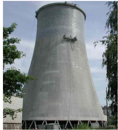
Winding the SikaWrap®-200 C carbon fibre reinforced fabric (width: 15 cm), centre-to-centre distance 30 cm.
