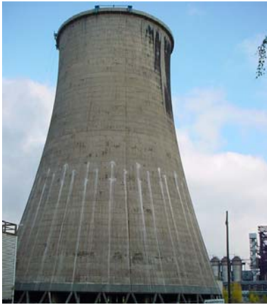
Quality control of the concrete. Core drilling on the wall.
