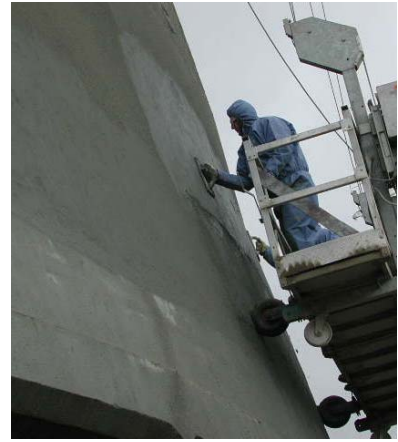
Finishing the SikaCem®-Gunit® 212 S after spraying.
