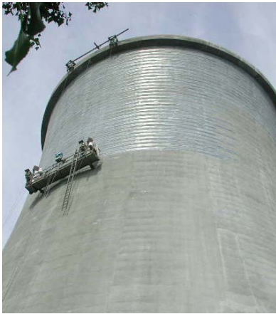
Winding the SikaWrap®-200 C carbon fibre reinforced fabric (width: 15 cm), centre-to-centre distance 30 cm.
